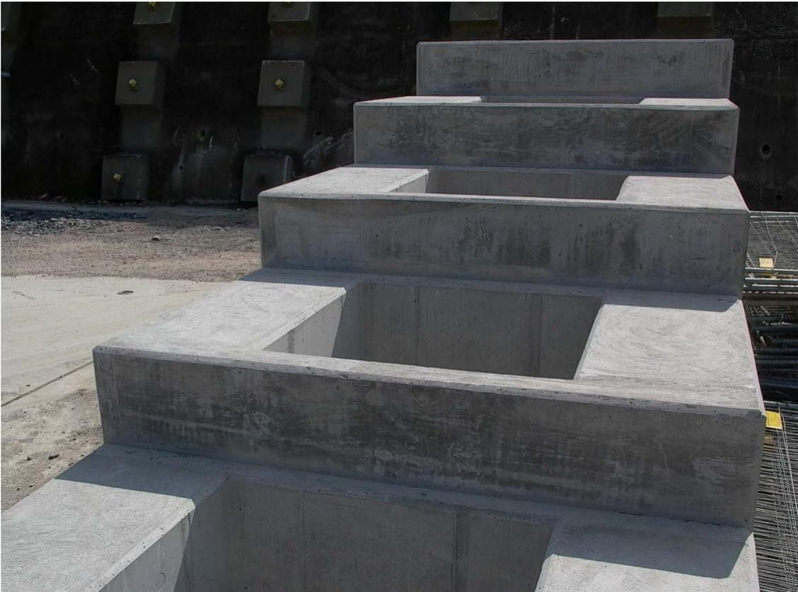
Top view of the exhaust shafts for the installation of the extract fans and dampers (20 May 2004).
