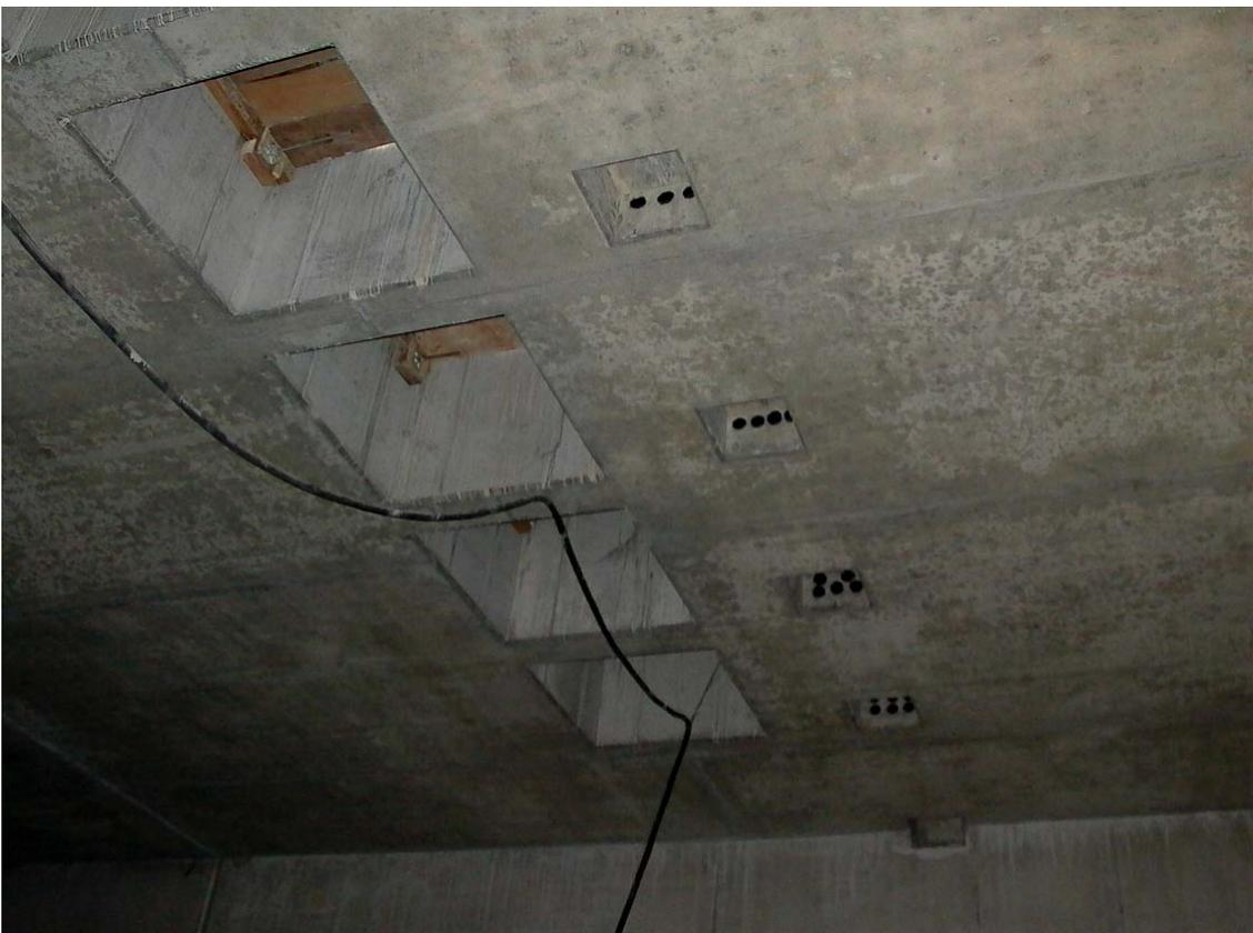
Bottom view of the shafts and holes for the installation of the extract fans and cables (20. May 2004).
